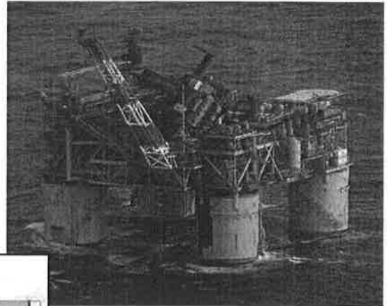
Mars Tension-leg Platform showing damage from Hurricane Katrina (2005)
